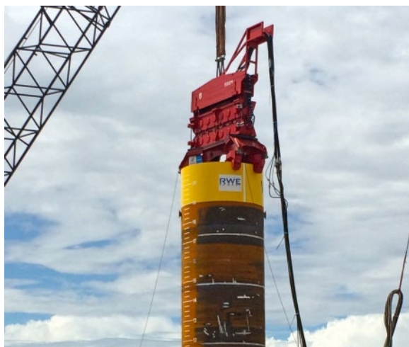
Figure 2-2: Example casing, with vibro-hammer.
