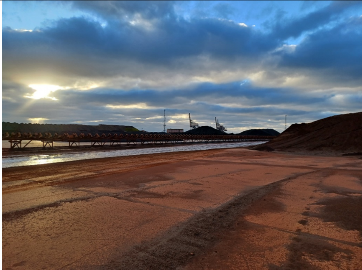
Image 2: View of Primary Ore Stockyards.
