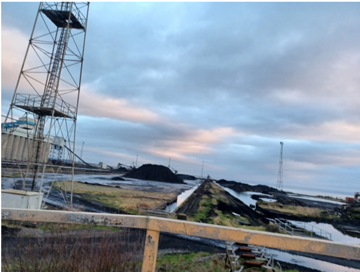
Image 7: View of Morfa Stockyards (Primary Coal Stockyards)
