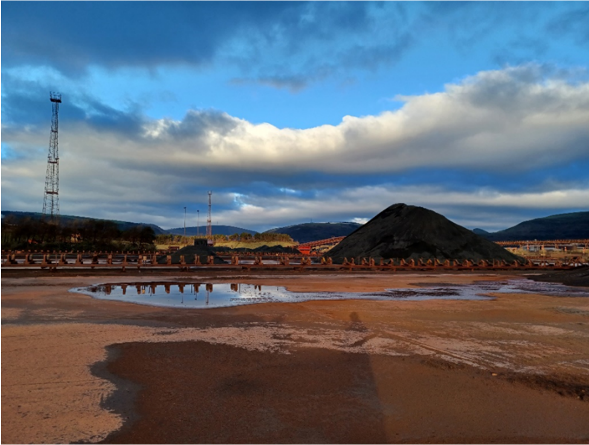
Image 1: View of Primary Ore Stockyards
