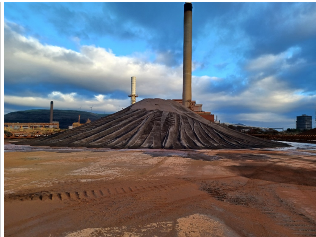
Image 3: View of Primary Ore Stockyards.
