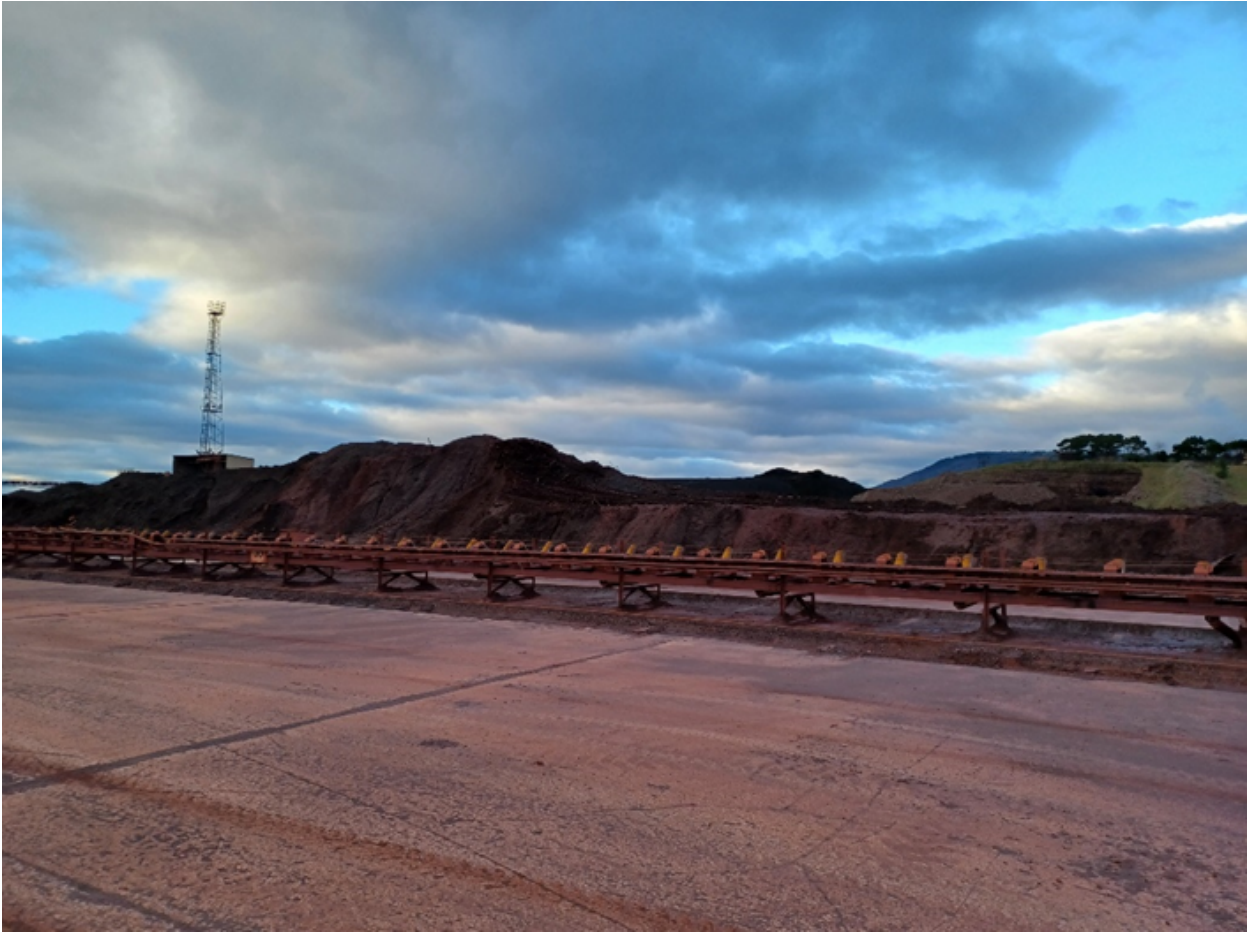
Image 4: View of Secondary Ore Stockyards
