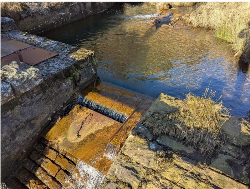
The Intake at the Nant Carnfeosen and Nant Melyn was also clear, with water passing over both the intake and the compensation notch.
