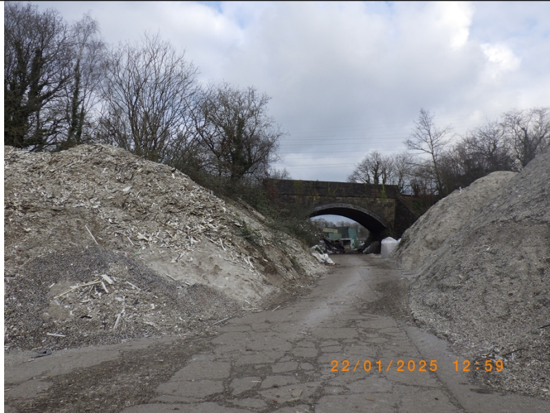
Image (4) of waste storage at the rear of the site
