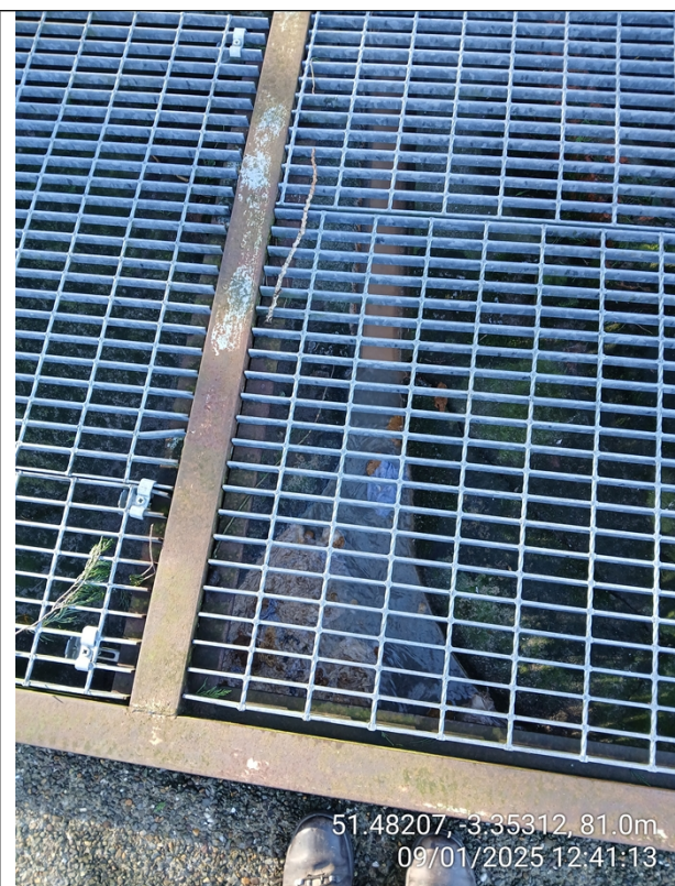
Inlet channel at site
