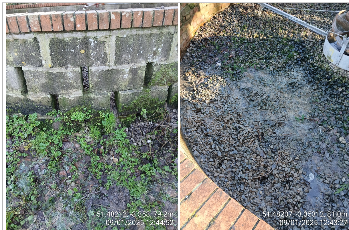
Left: Gaps between breeze block in filter bed 1.
