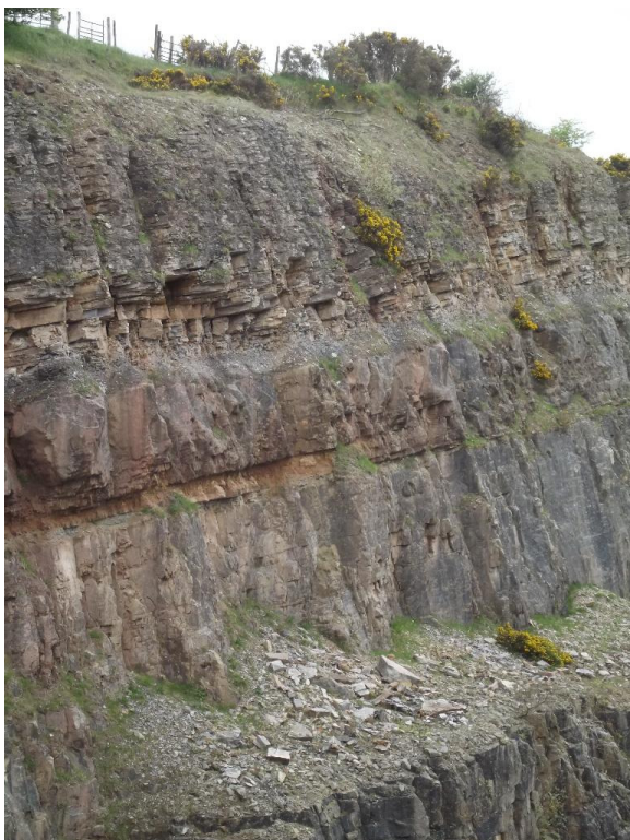
Plate 13: Failed rock forming scree on bench (note close proximity of boundary fence at this location).
