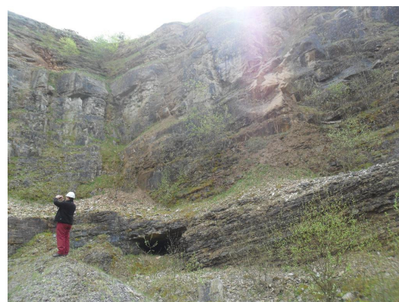
Plate 7: Potential wedge and planar failures in southern (northerly facing) slope.
