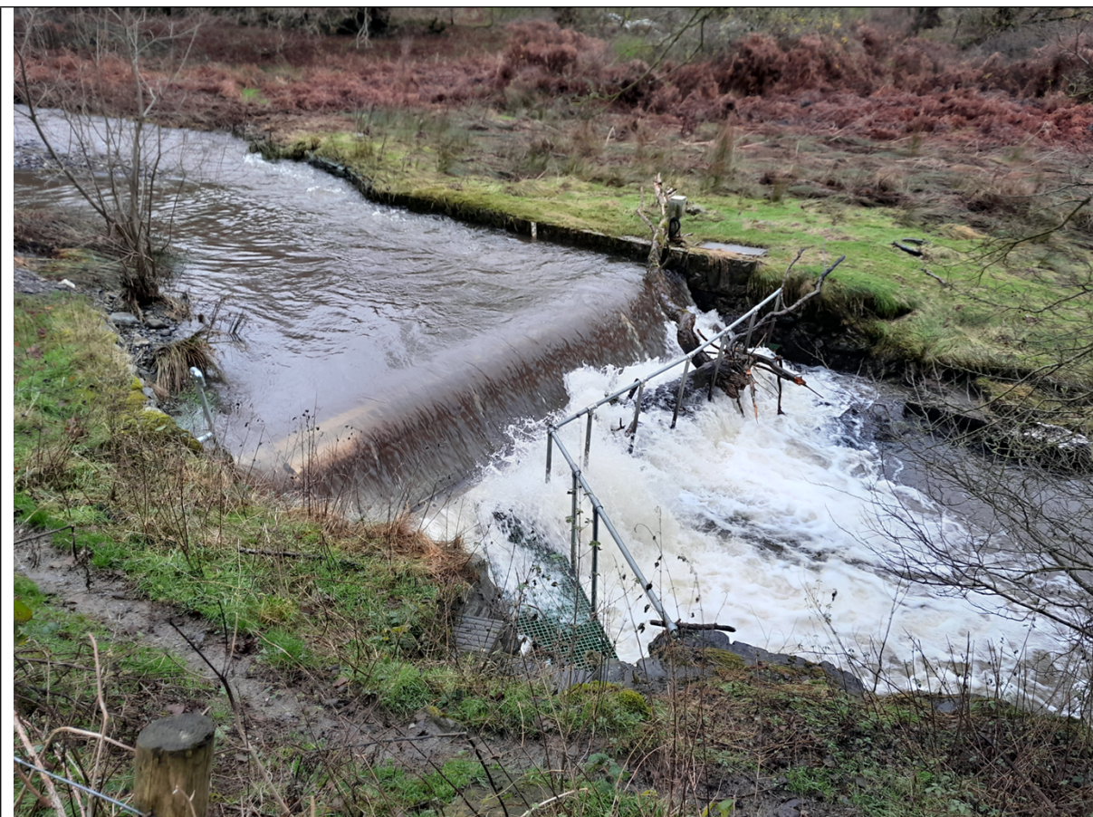
Photo 1. Impoundment overview, high flow, algae on coander screen, woody debris snagged by railings.
