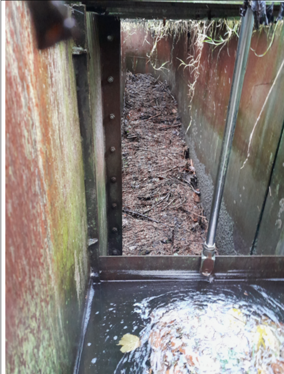
Photo 3. Sluice gates shut and debris collected in the screen box.
