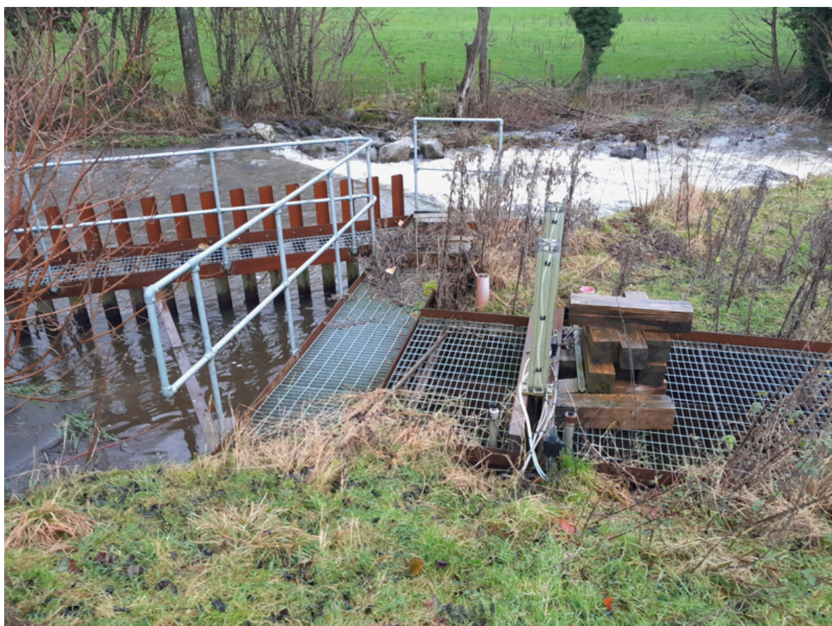
Photo 1. Overview of the impoundment infrastructure
