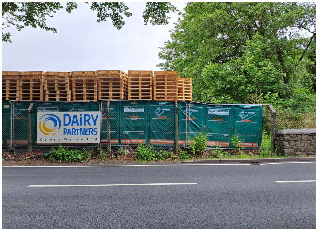
Figure 1 - Site boundary fence with acoustic paneling/barrier and wood pallets.
