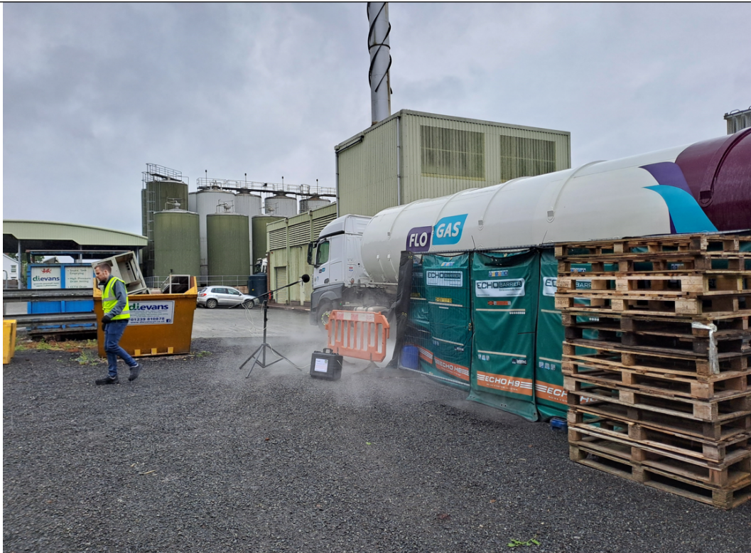
Figure 2 - LNG delivery with acoustic paneling/barrier and wood pallets.
