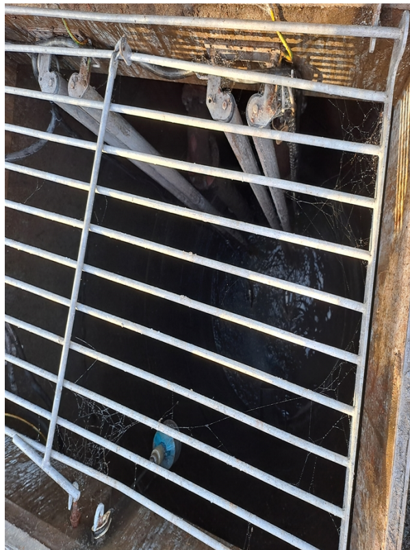
Figure 3: Site visit photo – The wet well as observed during the visit.
