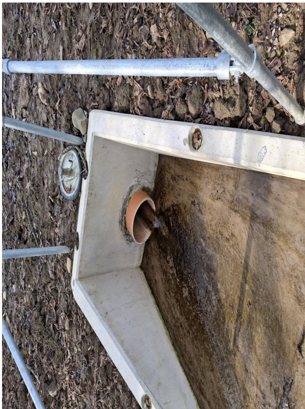
Figure 2: Clear water discharging from discharge point 2
