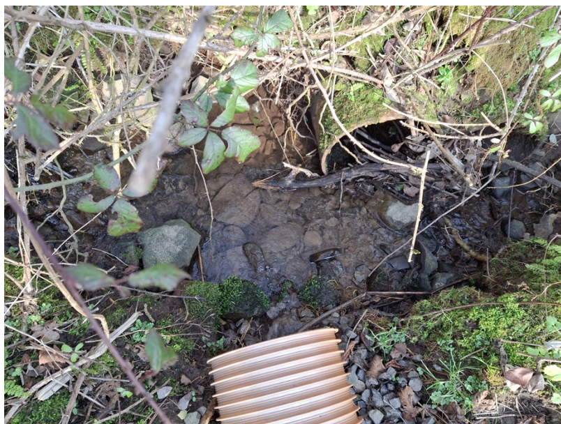
Figure 4: Clear water discharging from discharge point 4
