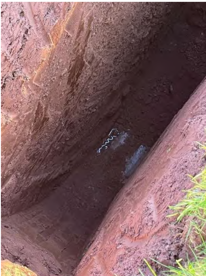
Figure 2-7 TP02 minor water seepage
