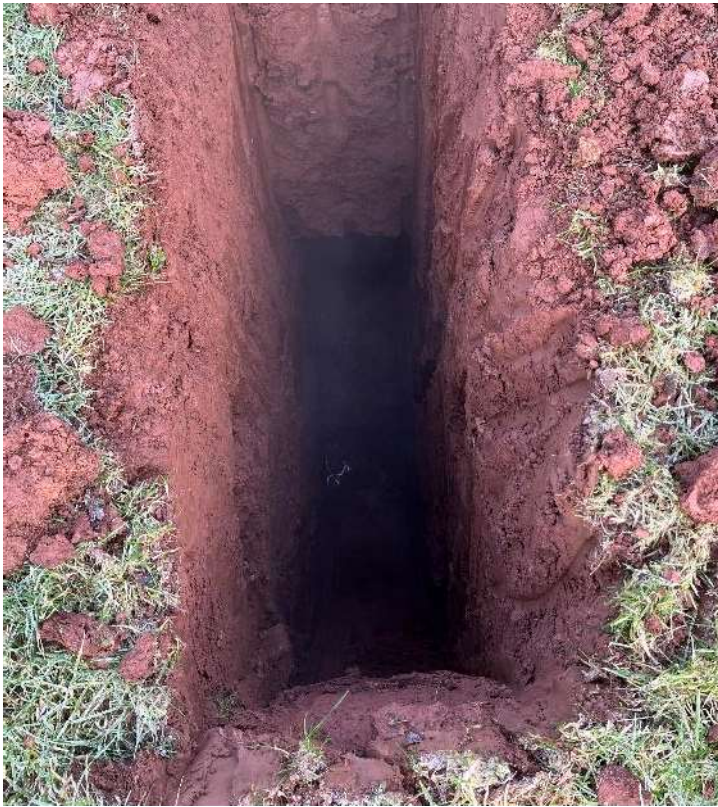
Figure 2-3 TP01 start of water seepage
