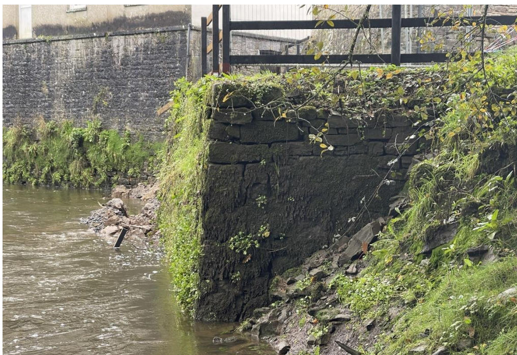
Figure 3. Surviving section of wharf wall, showing its rubble-stone construction.
