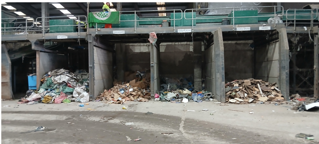
Photo 3 - View inside waste transfer station building sorting bays
