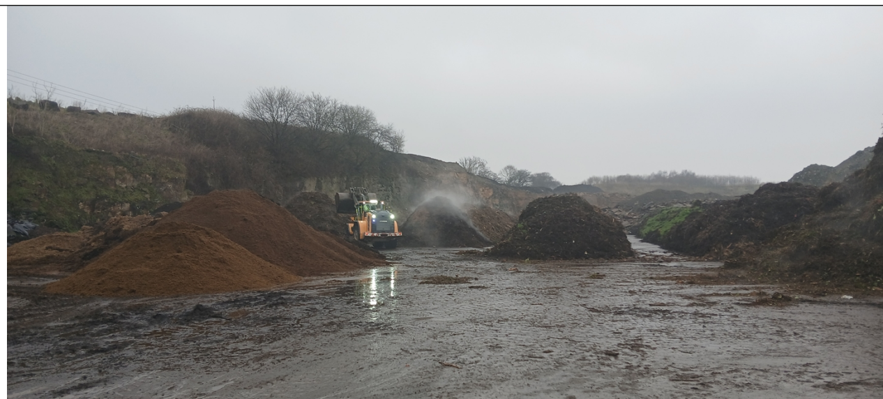
Photo 8 - View of the composting station area
