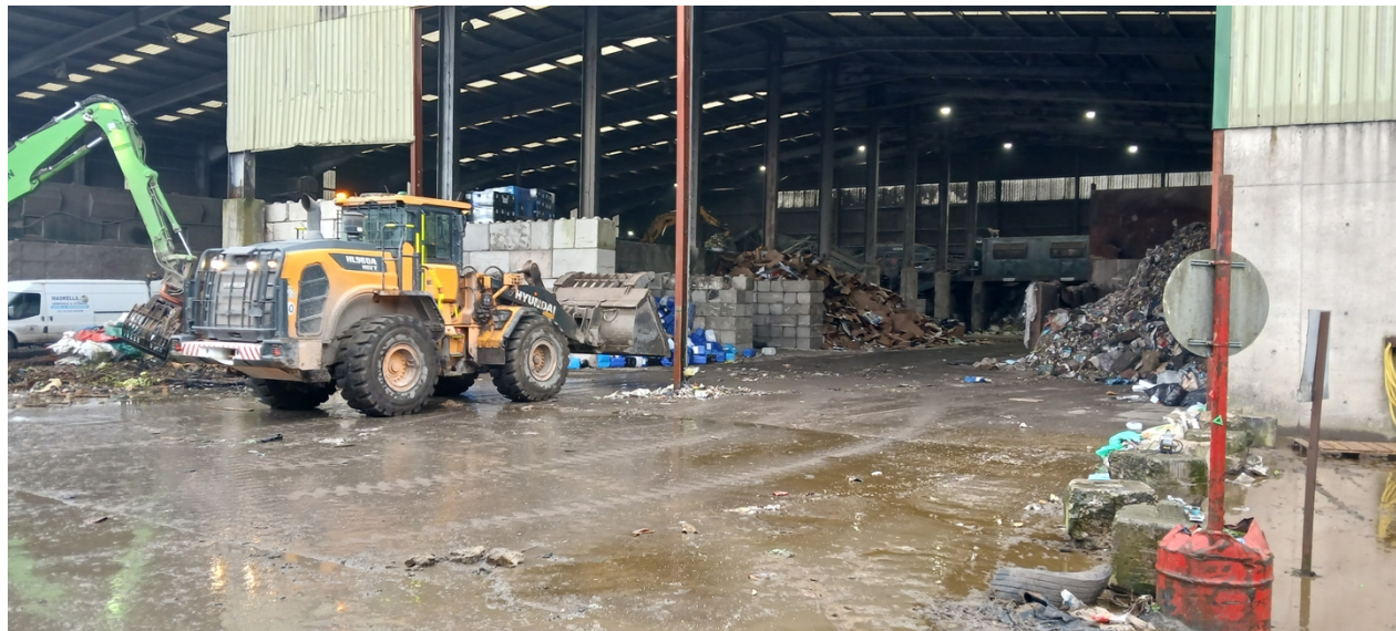
Photo 1 - View inside waste transfer station building
