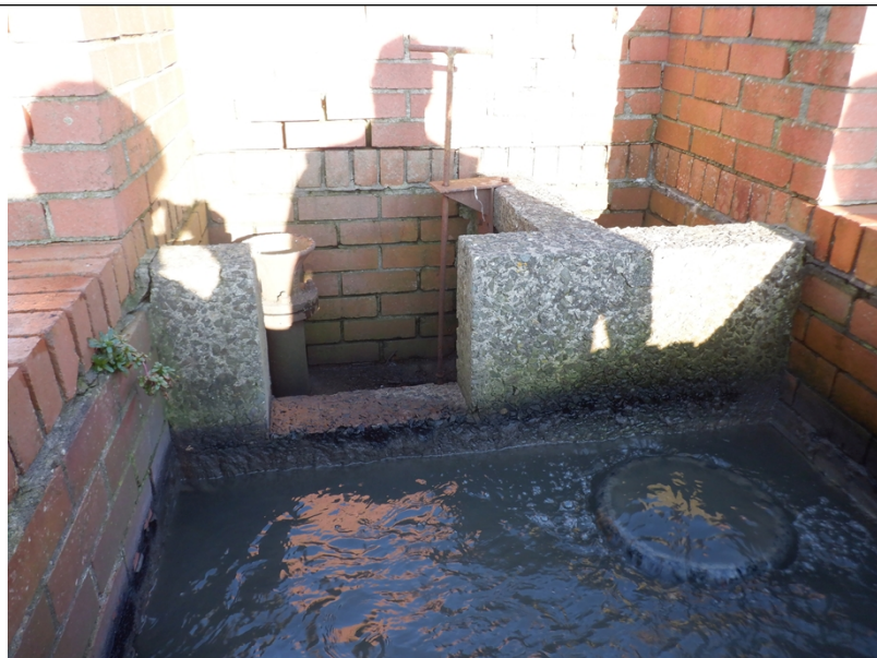
Image1. Showing overflow weir that could allow discharge outside of permit conditions.
