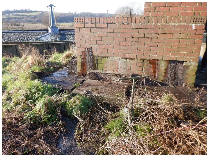
Image 2. Showing leak of sewage from flow splitting chamber.
