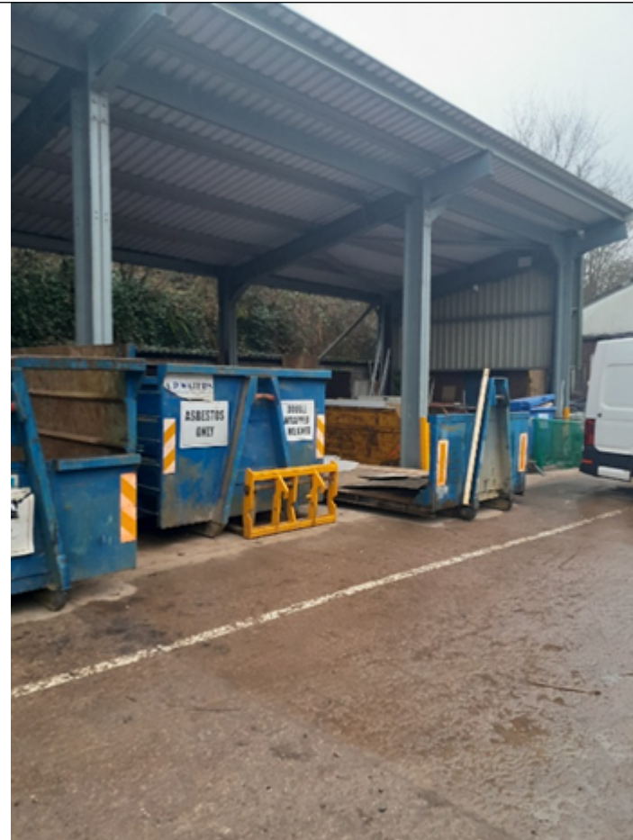
Image 1 showing separated skips with the different waste streams stored within building.
