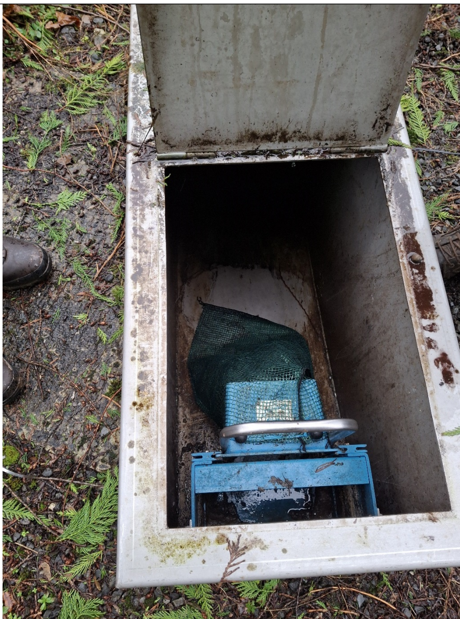
Figure 1. Copa Sac on the storm discharge, not in operation at the time of the inspection.
