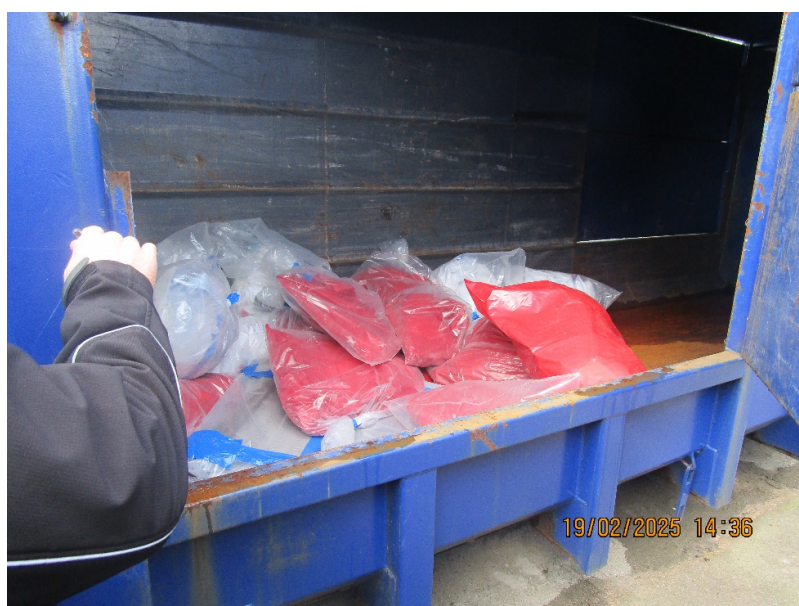
Figure 2. Fibrous asbestos skip containing asbestos waste double bagged.
