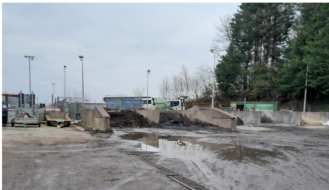
Figure 2 : shows pooling caused by blocked drain.
