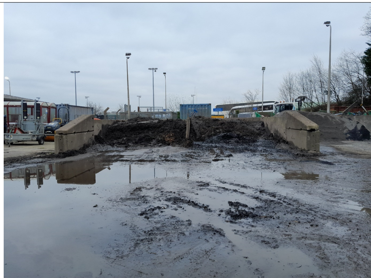
Figure 3: shows pooling on the impermeable pavement from another angle.
