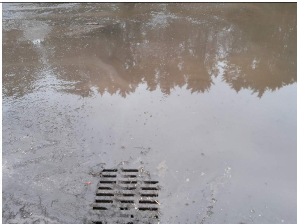
Figure 1: shows blocked drain.
