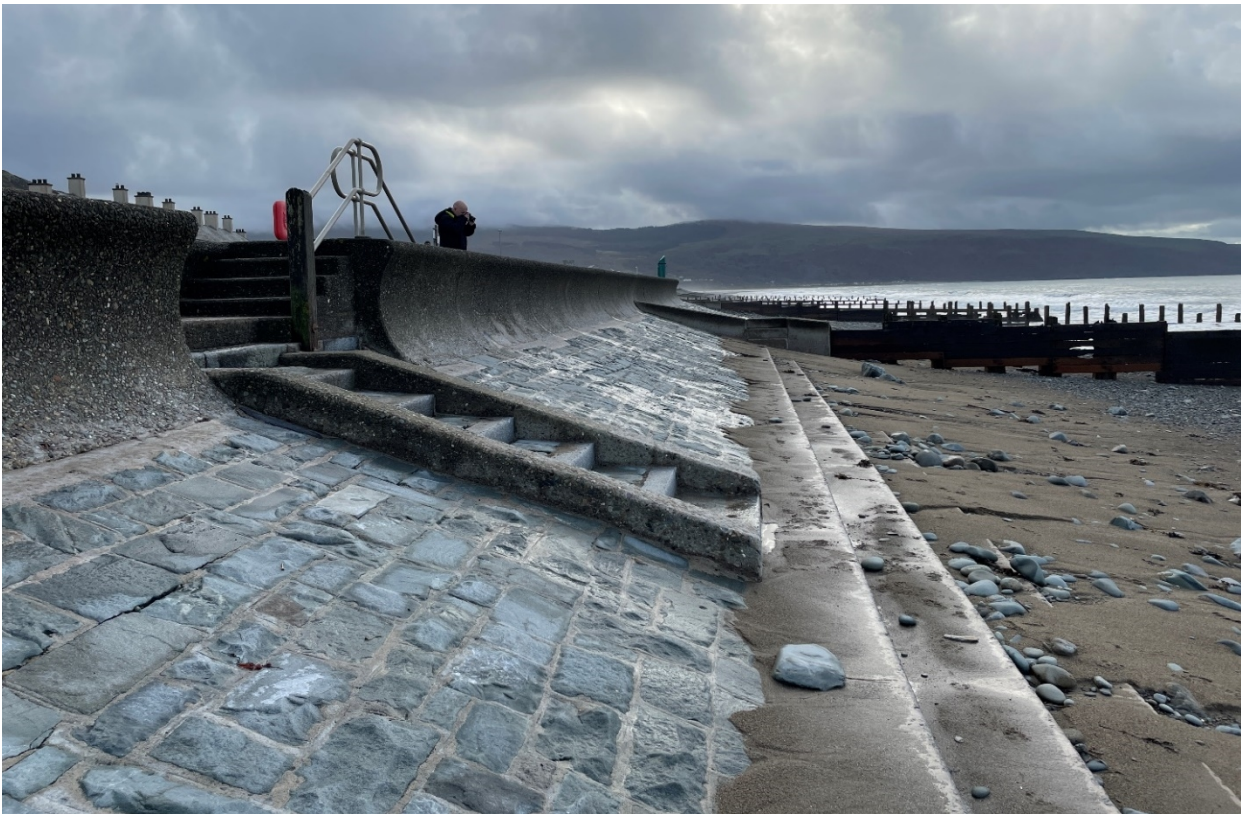
Photograph 7 View south showing the 1930s stone-faced apron wall and stone steps, 1930s concrete stepped sea wall, and 1970s wave return wall
