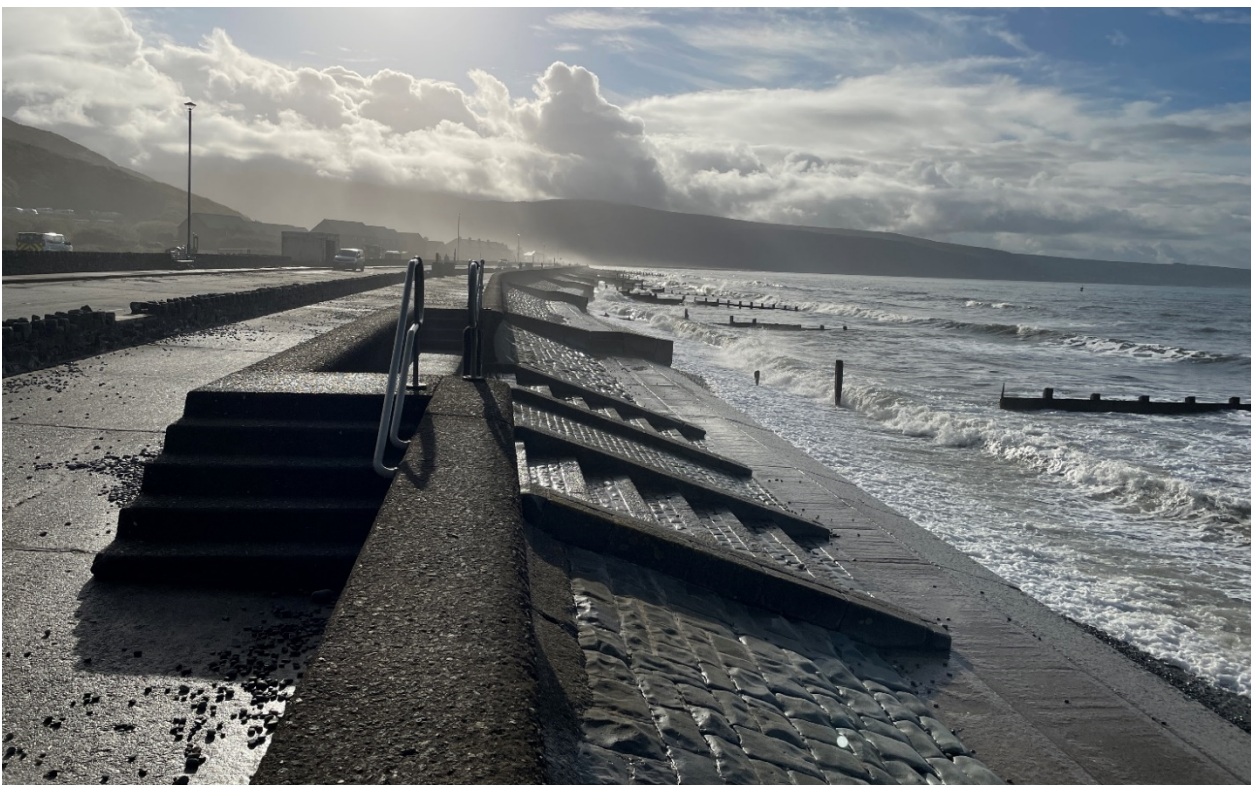
Photograph 8 View south showing the 1930s stone-faced apron wall and stone steps, 1930s concrete stepped sea wall, and 1970s wave return wall
