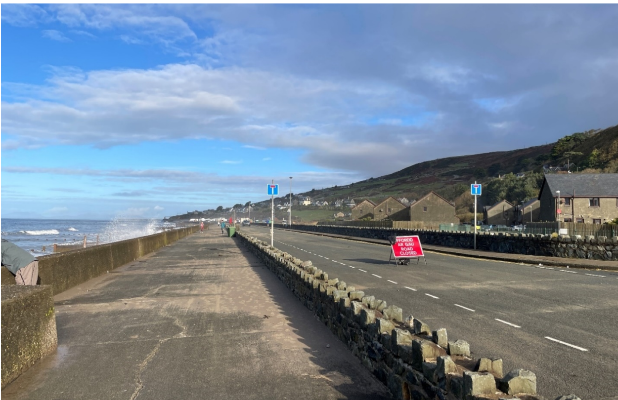
Photograph 2 View north along the promenade, showing the stone wall (centre) dividing the promenade and roadway, and the 1970s wave return wall (left)
