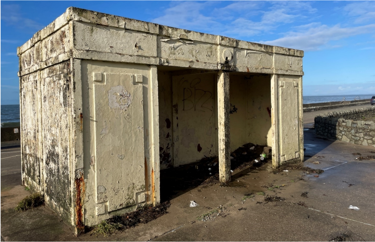
Photograph 11 View west of rear of rain shelter
