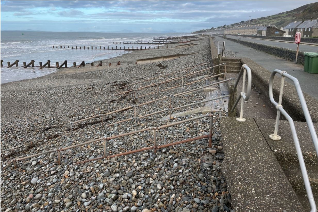
Photograph 3 View north along the beachfront, showing the 1970s wave return wall, timber groynes, and shingle covering the 1930s stone-faced apron wall and steps down to the beach
