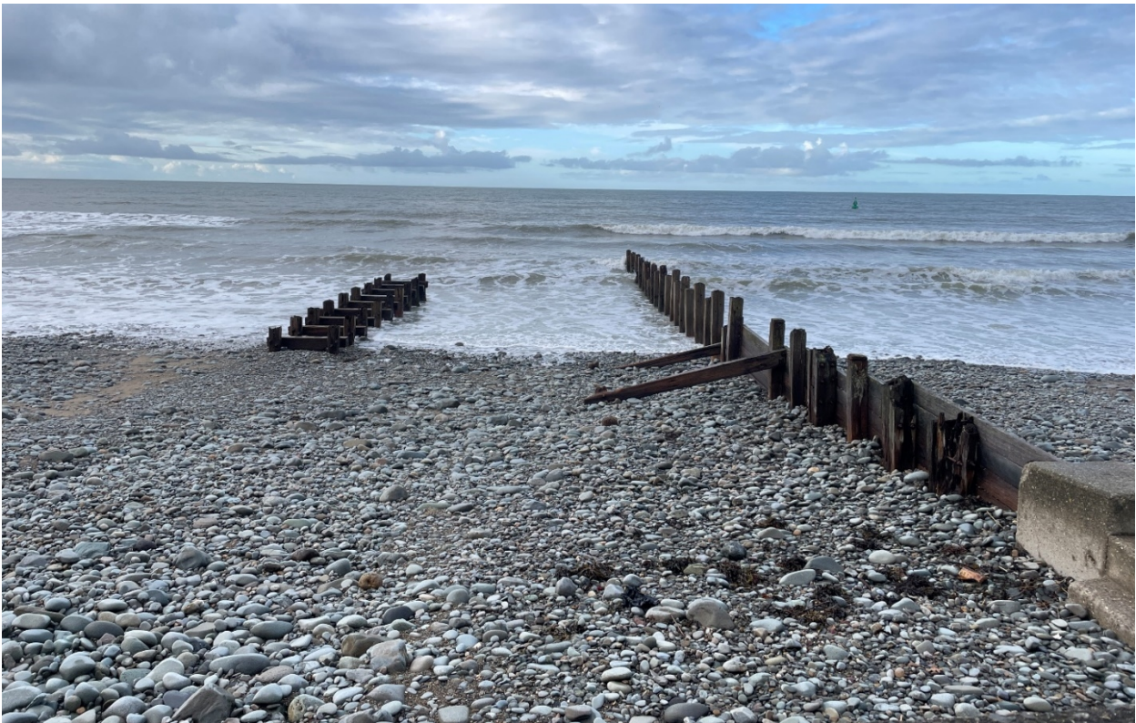
Photograph 5 View west showing timber groyne (right) and timber cradle (left)
