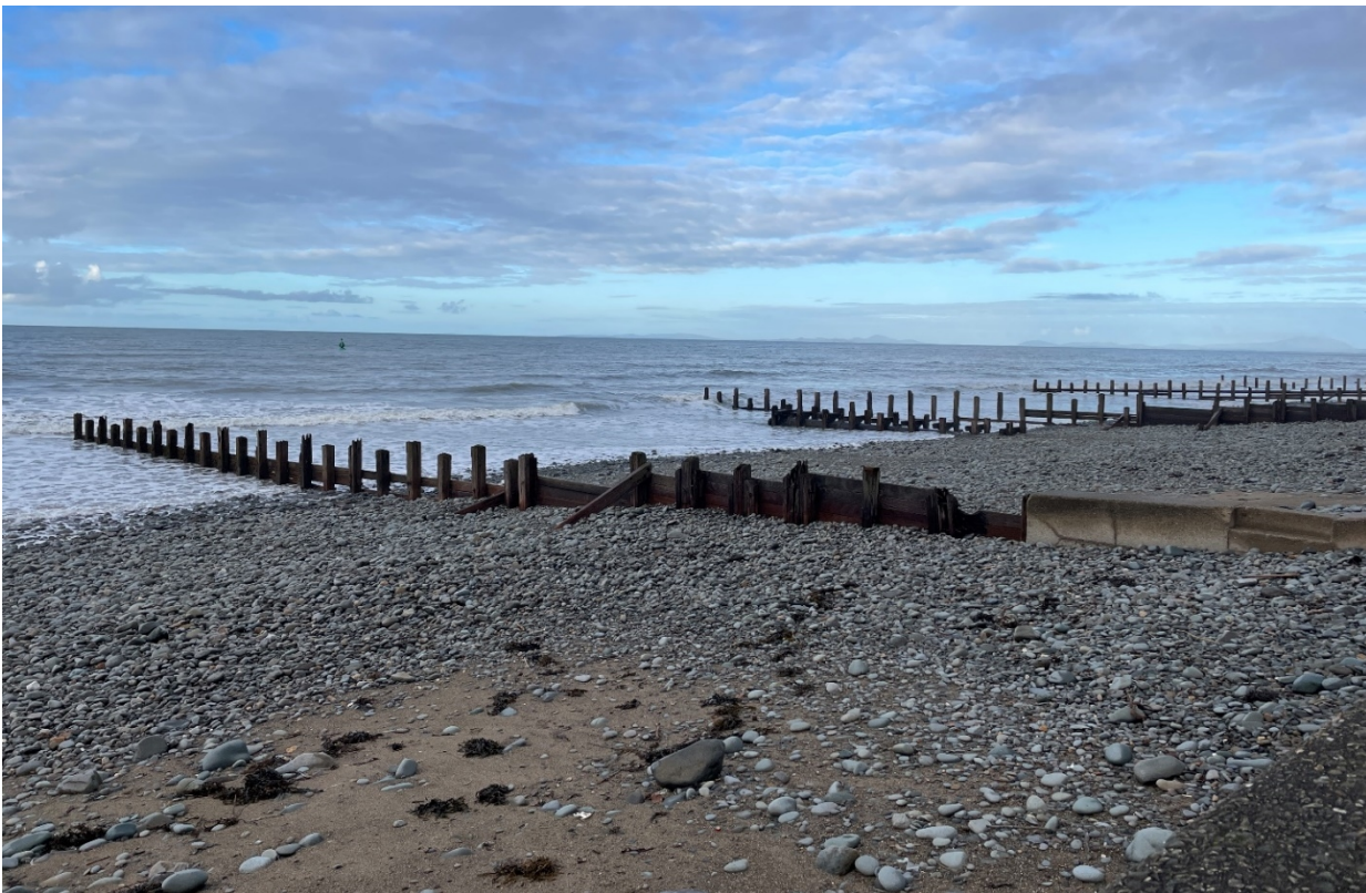
Photograph 4 View northwest showing the beach and timber groynes
