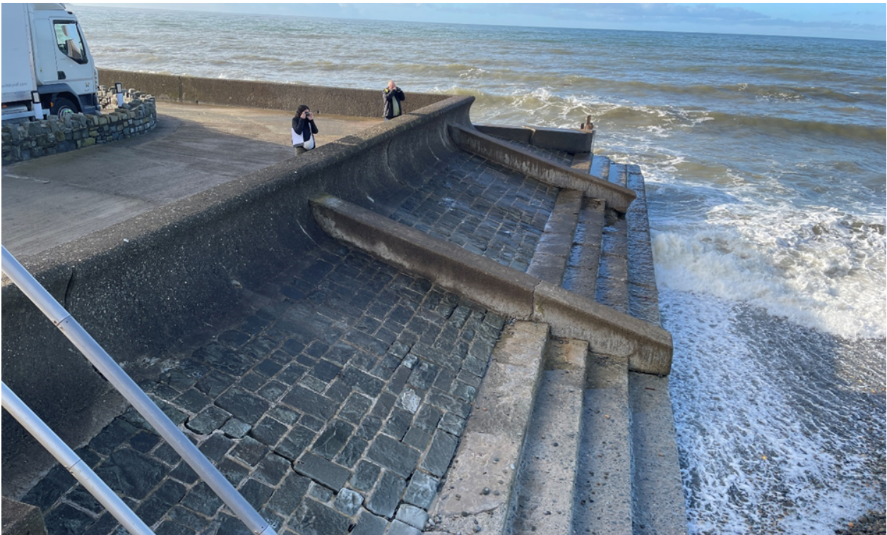
Photograph 9 View west showing the northern end of the 1930s sea defences, with 1930s stone-faced apron wall and concrete stepped sea wall, and 1970s wave return wall
