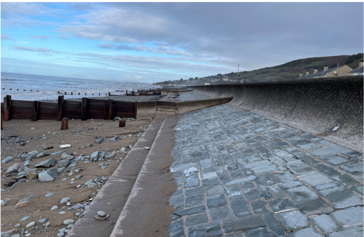
Photograph 6 View north showing the 1930s stone-faced apron wall
