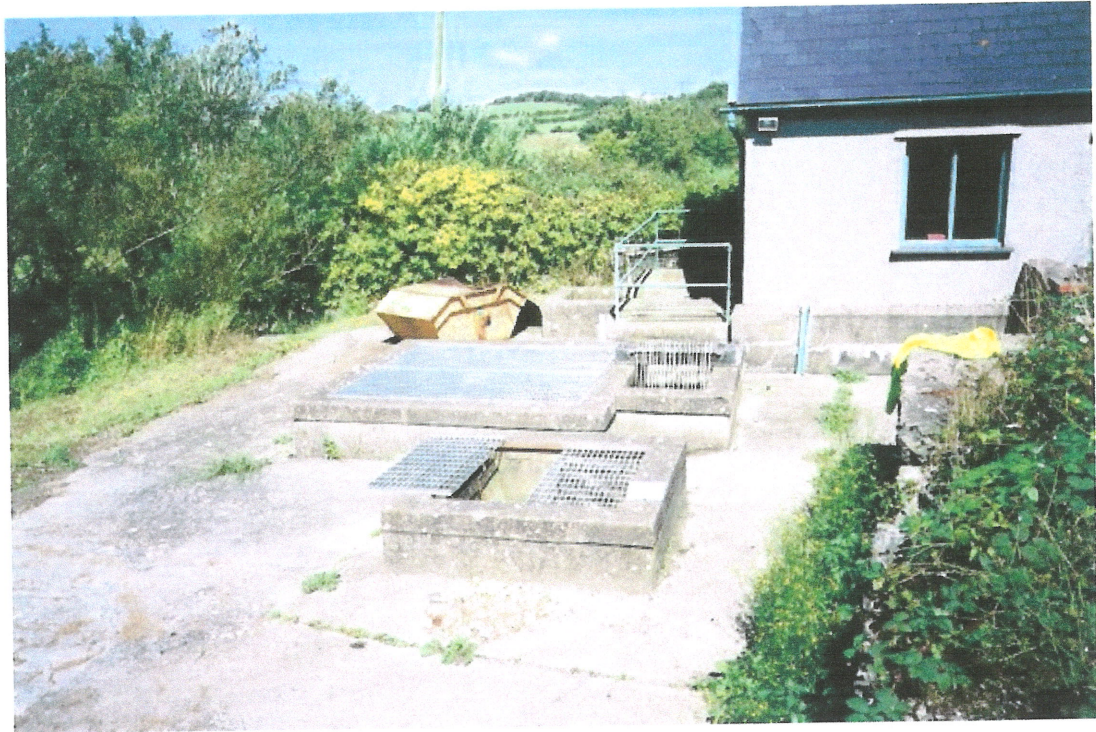
Photograph No.2 - Plan view of bifurcation chamber and macerator /screening chamber
