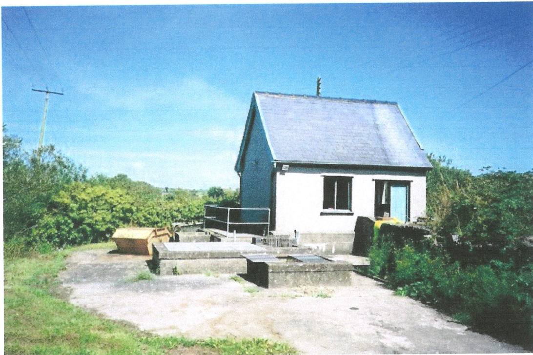
Photograph No.1 - Bodedern Pumping Station Compound
