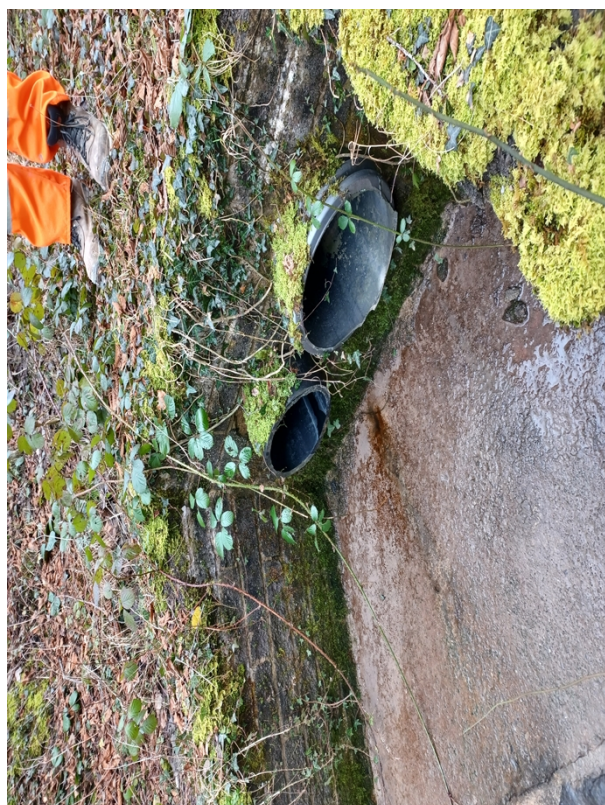
Figure 3: Outfall location. Left pipe is discharge from void, right pipe is storm discharge.
