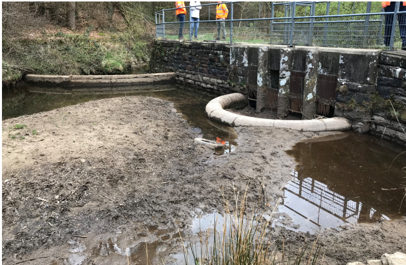
Photo of head of bywash (left) and inlet structure
