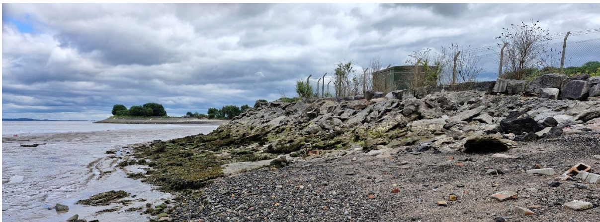
Image 6. View (southeast) of the northwestern part of remedial area
