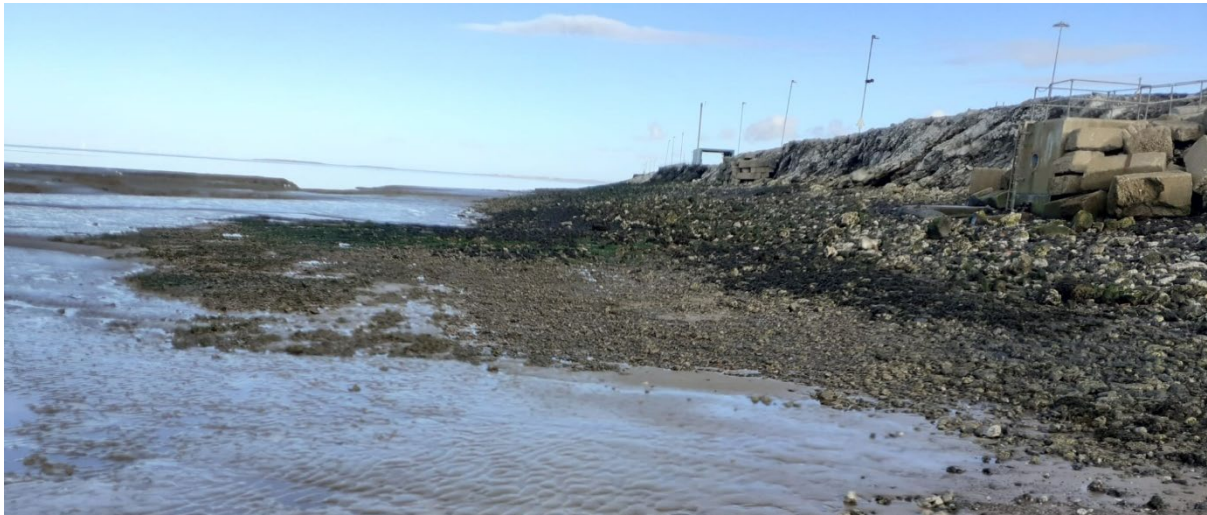
Image 2. View (northeast) of the central part of scrape back area
