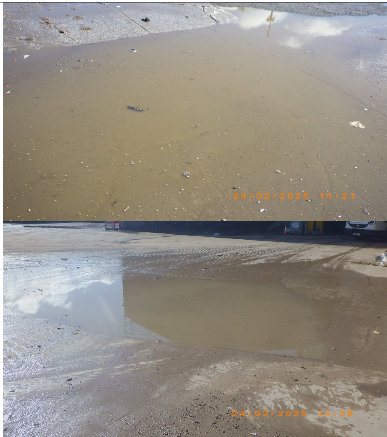
Photos showing standing water and blocked drains on site
