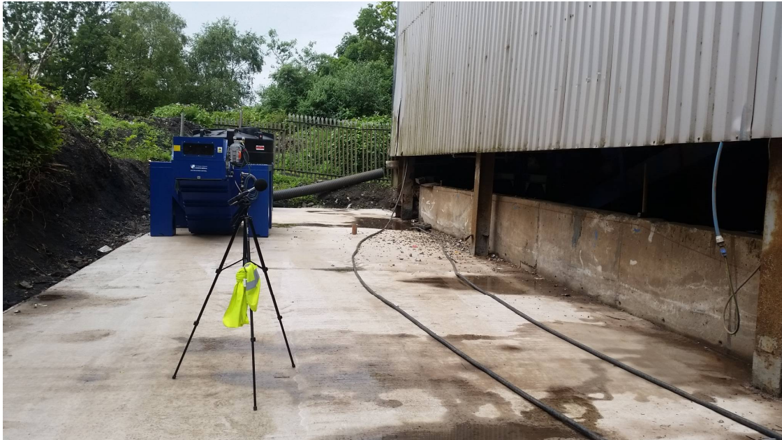
Picture 5A: gap at the bottom of the recycling building to be repaired and sealed to reduce the break out of noise.
