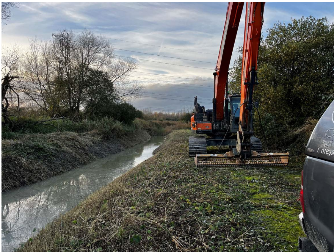
Plate 3-7 Ongoing clearance of inner ditch south of Lagoon 25 (12 November 2024)
