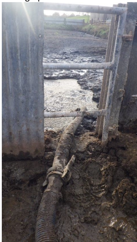
Photograph of pipe to farm lagoon from which tanker was being filled.
