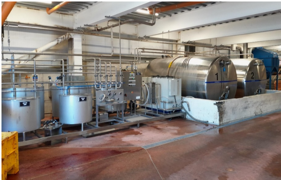
Image 2 – showing blood tanks and refrigeration systems, taken on 3 October 2024
