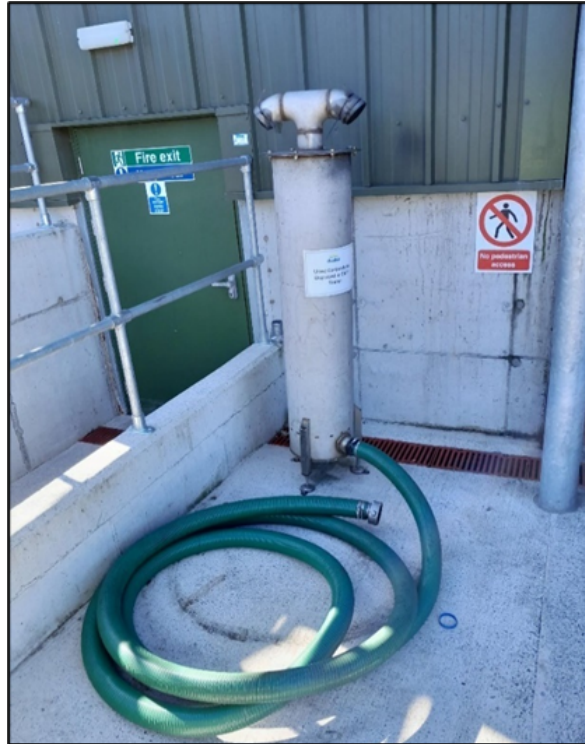
Image 3 – showing carbon filter outside the blood storage unit, taken on 3 October 2024
