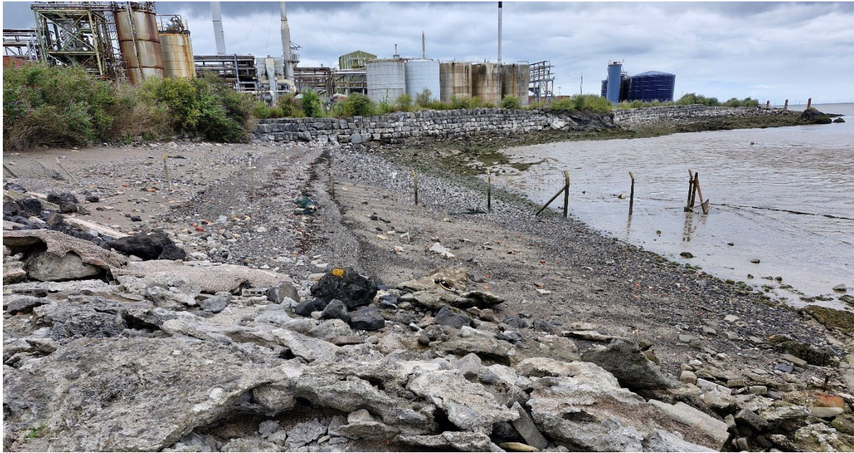
Image 7. View (northwest) of the northwestern part of remedial area
