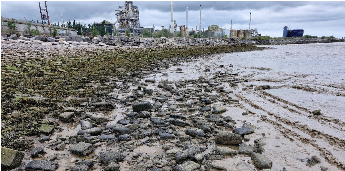
Image 5. View (northwest) of the central part of remedial area
