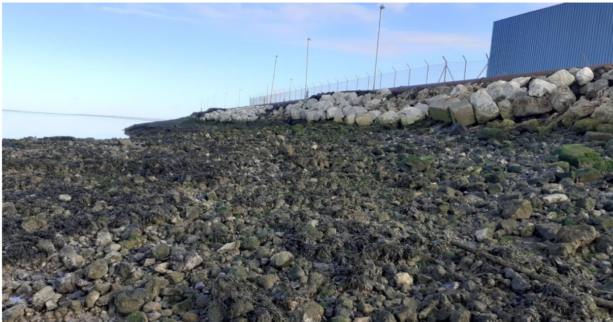
Image 3. View (northeast) of the northeast part of scrape back area
