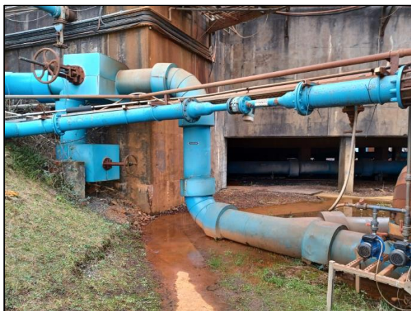
Image 5 and Image 4 – effluent pooling at clarifiers
