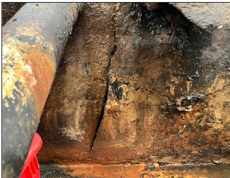
Image 2 – Crack in flume wall
