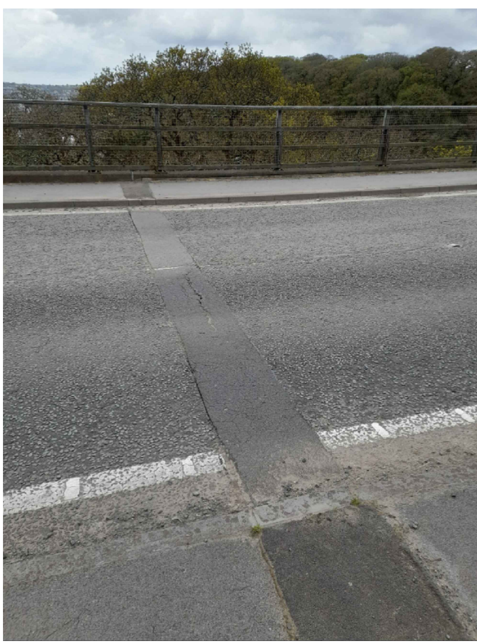
EXISTING ASPHALT PLUG
