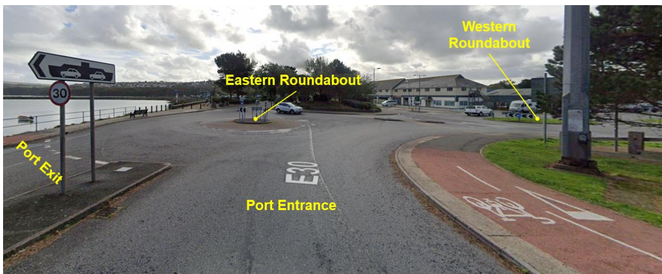
Figure 19.2: Illustration of Existing Port Roundabout Access (Google Maps)
