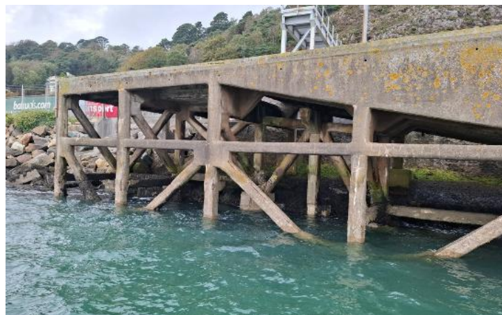
Figure 2-6 Disused RNLI Slipway Structure
