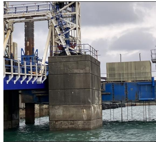
Figure 2-8 South Buffer Dolphin and Linkspan Tower Bridge
