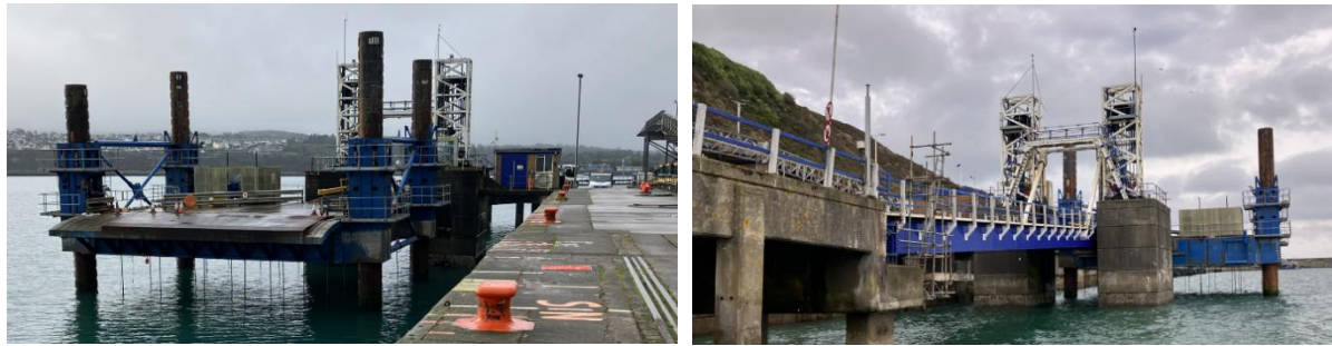
Figure 2-2 Existing Jack Up Barge, Linkspan Bridge, Towers and Concrete Buffer Dolphin
