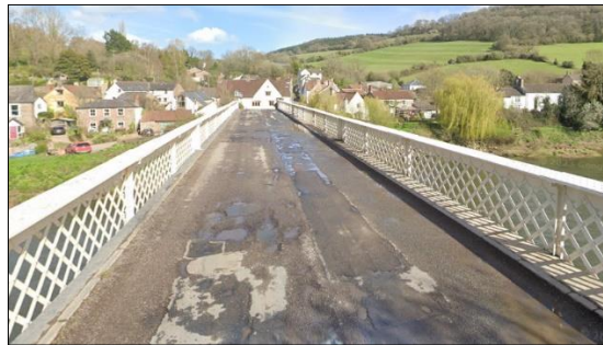
Figure 1: Brockweir Bridge Carriageway Surfacing
