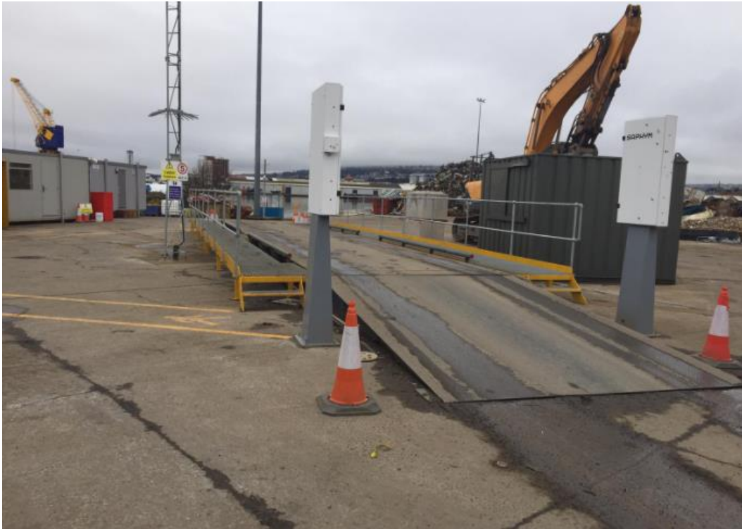
Photograph 3.4: Weighbridge and waste scanner within current area (March 2019)
