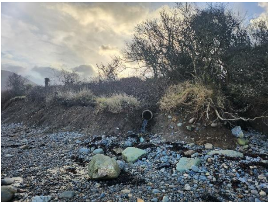
Site Photograph No 6 – Culverted unnamed watercourse outlet.
