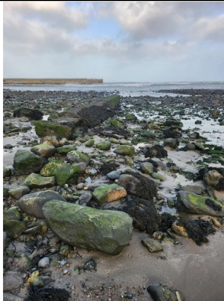
Channelled wrack was also attached to the broken drainage pipe.
