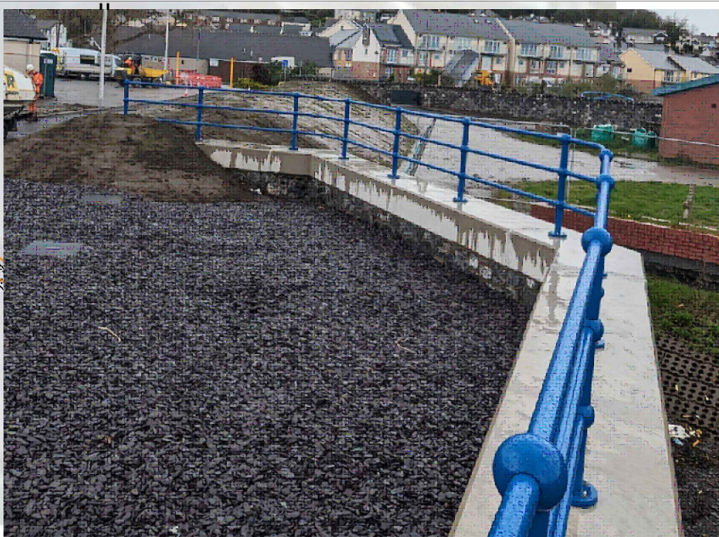
EXISTING SHEET PILES (VIEW FROM LANDSIDE)
