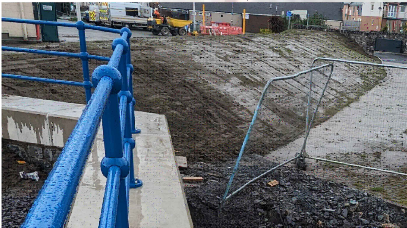
EXISTING FLOOD BUND
