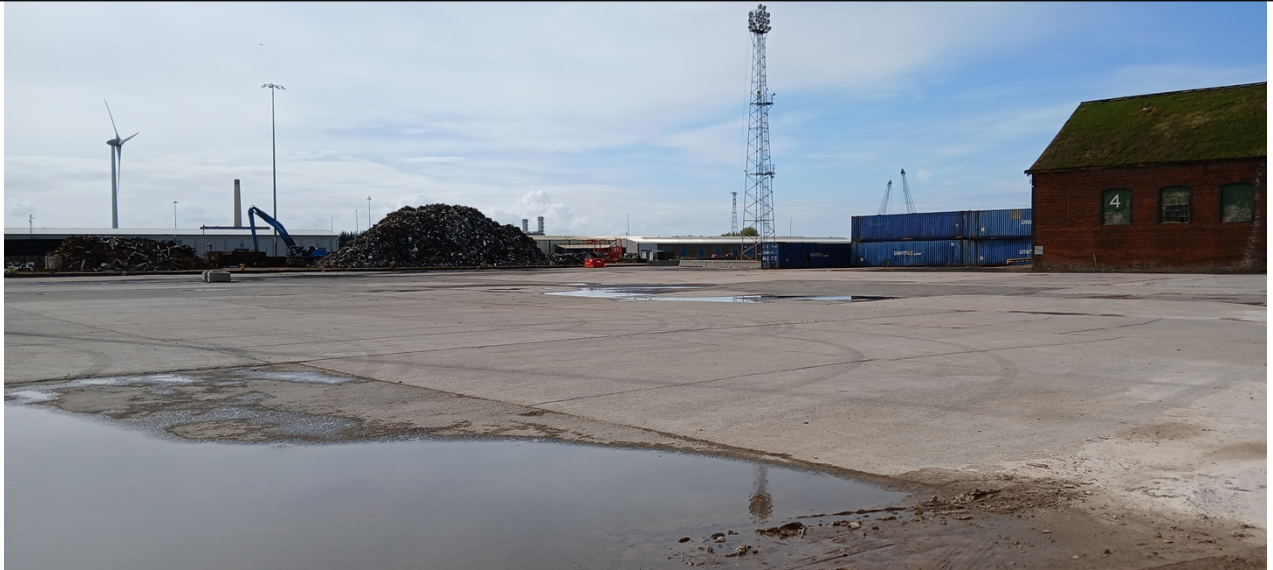
Photo 1 - SWWP Ltd Site, Alexandra Docks, Newport
