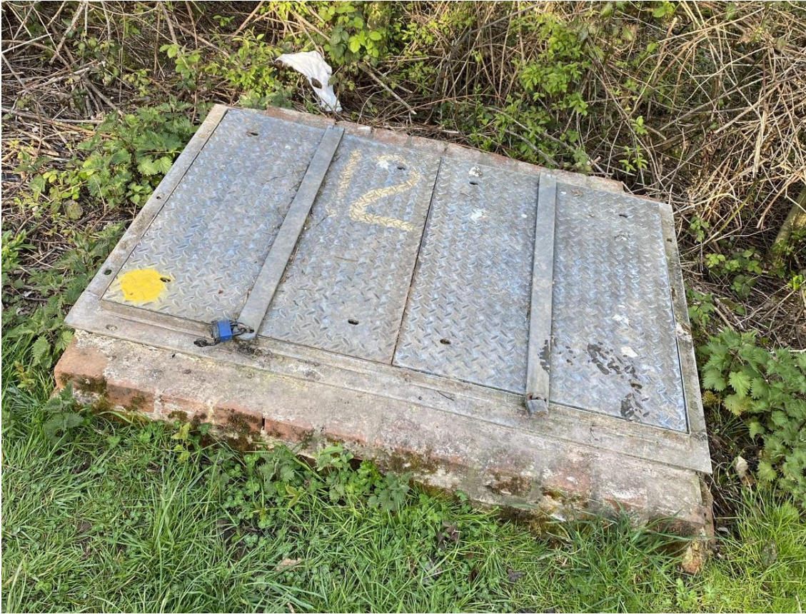
Figure 3.6: Leachate abstraction well LW12
