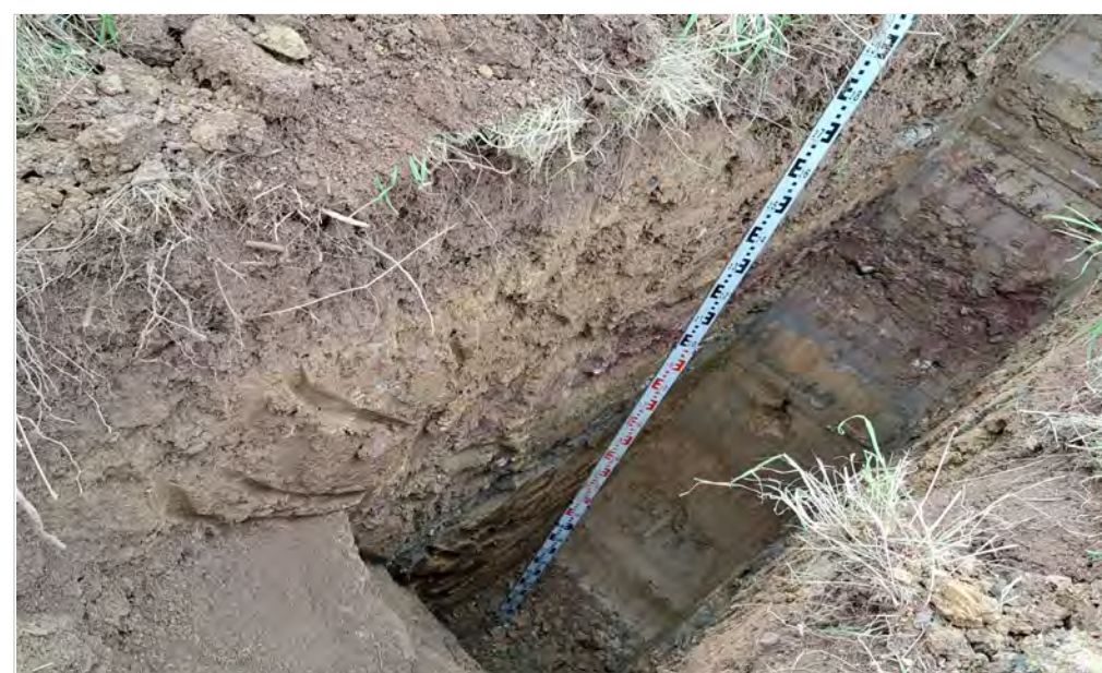
Plate 01: TP01 sidewall 0.00m to 3.10m
