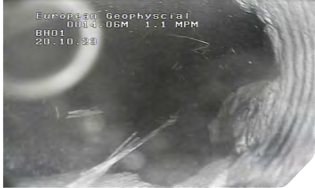
Plate 06: BH01 downhole view at 14.06 m bgl. Borehole walls visible on right hand side. Top of void.
