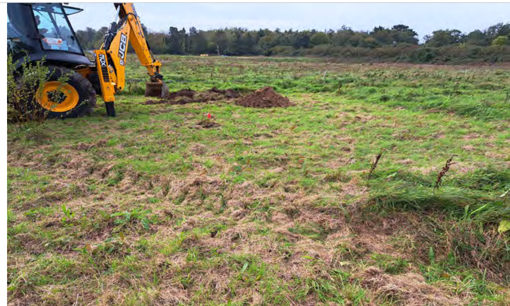
Plate 24: Trial Pitting at TP03.
