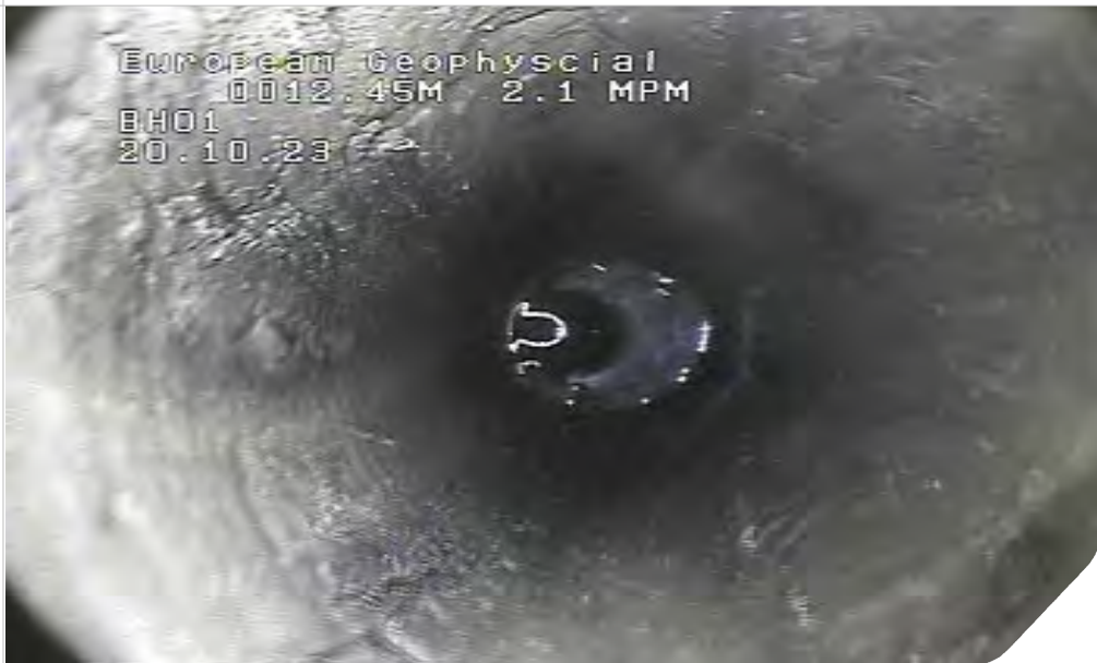
Plate 07 BH01 downhole view at 12.45 m bgl. Water table can be seen below. Regular borehole sidewalls.
