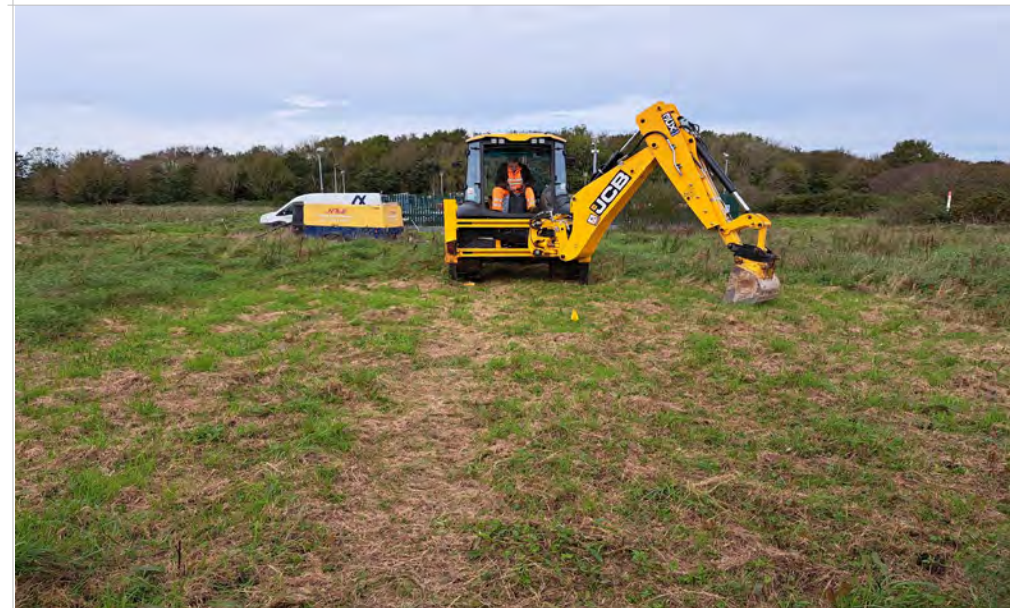
Plate 23: Trial Pitting at TP05.
