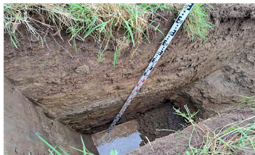
Plate 17: TP09 Sidewall 0.00m to 2.70m.
