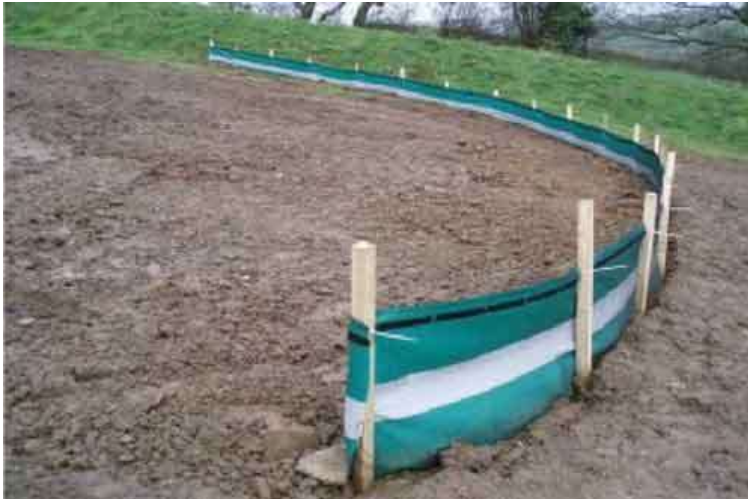
Typical silt Fence
