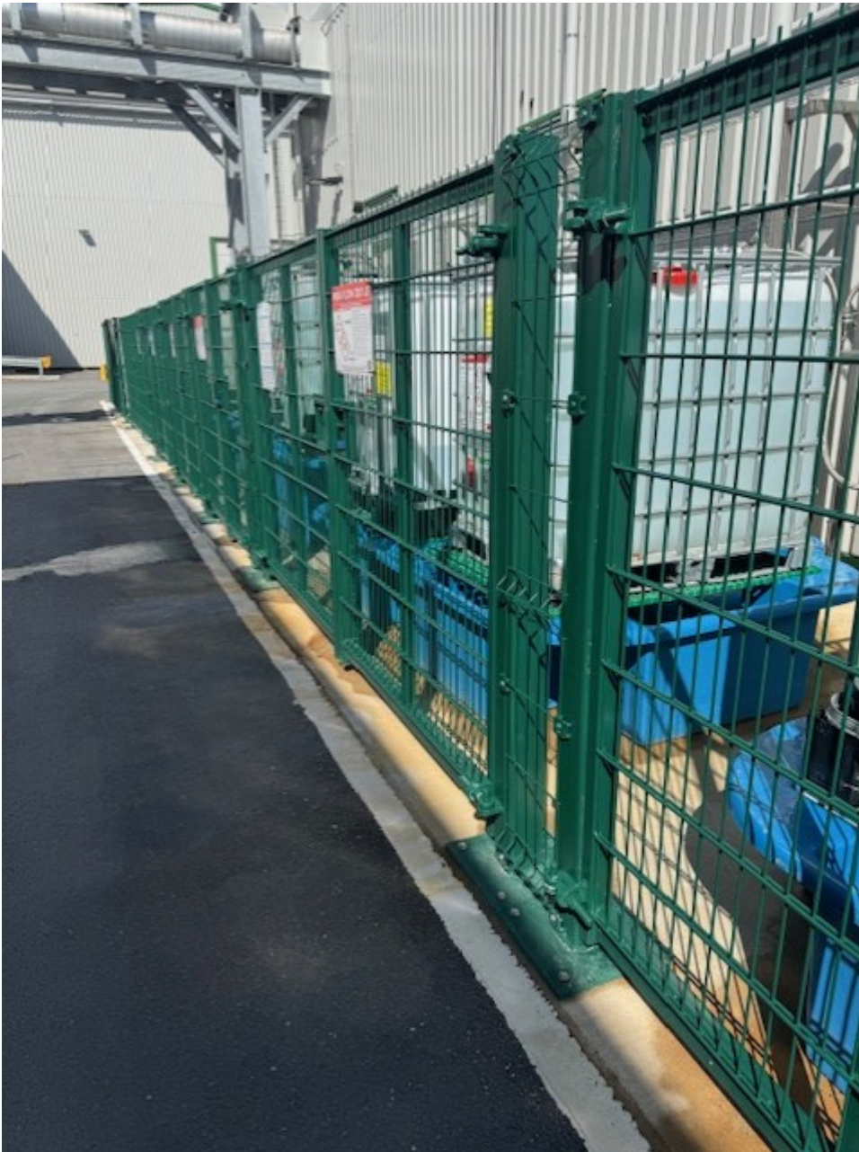
PHOTO 6 – No Lip on Storage Access Area
