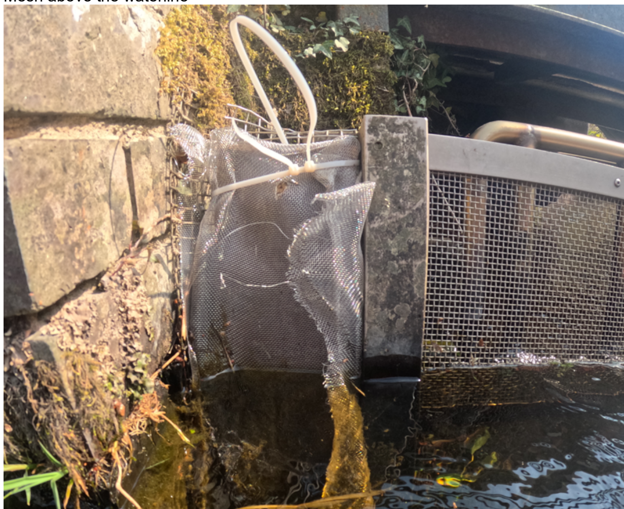
Mesh above the waterline
