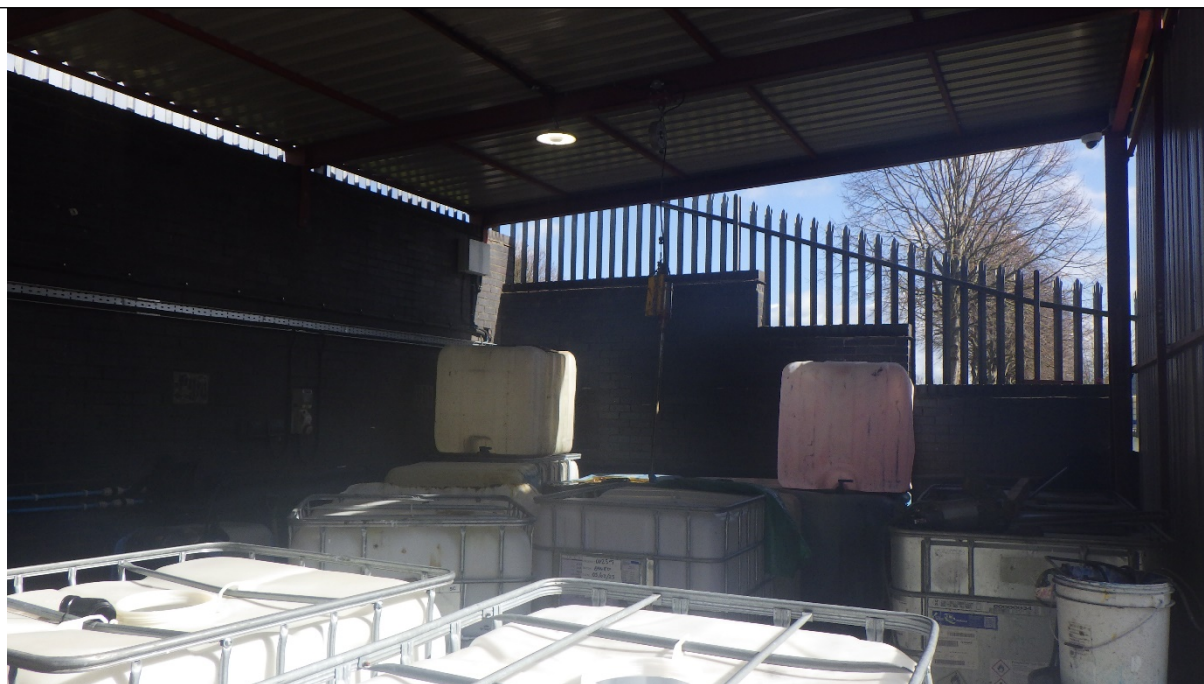
Outside IBC wash plant.
