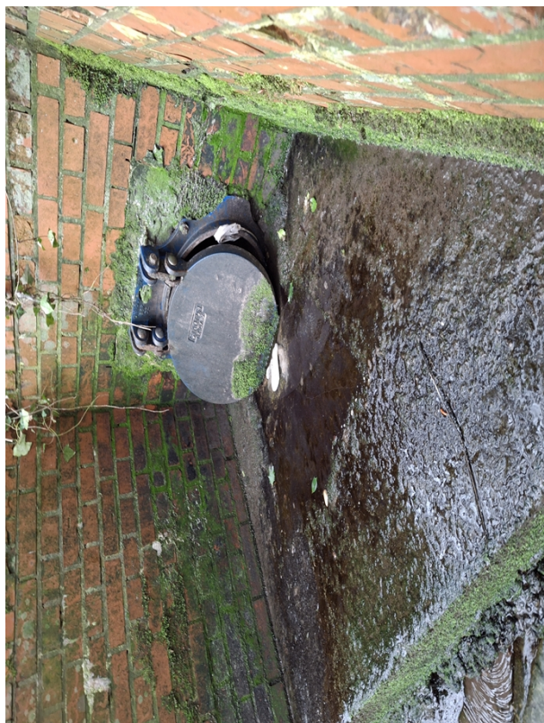
Figure 1: Slight ragging around discharge point
