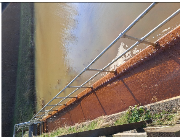
Figure 4 – Right hand outlet with significant sediment build up at the time of the visit.
