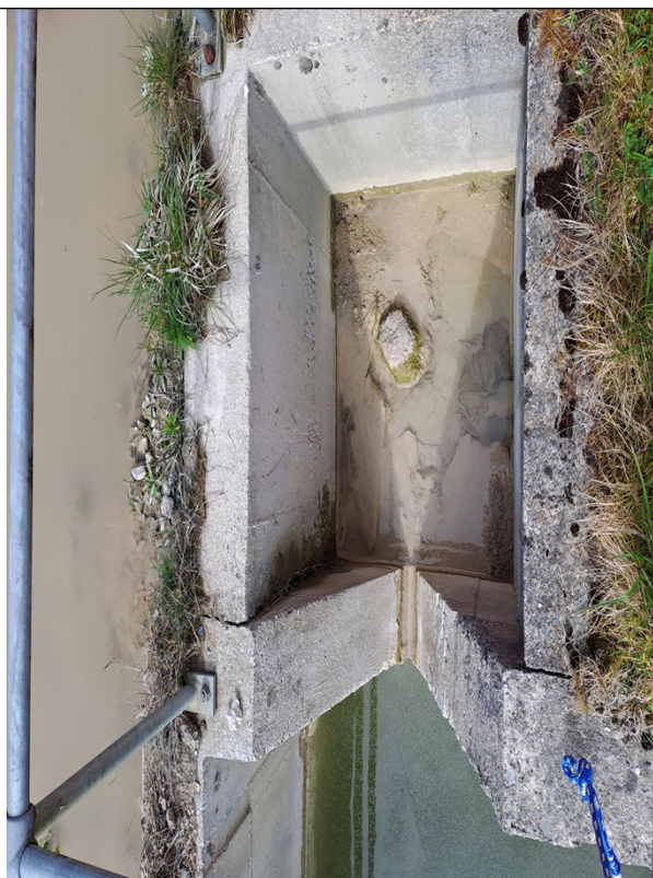
Figure 7 – The discharge point of the treatment tanks to the wider site drainage. No flow at the time of the visit.
