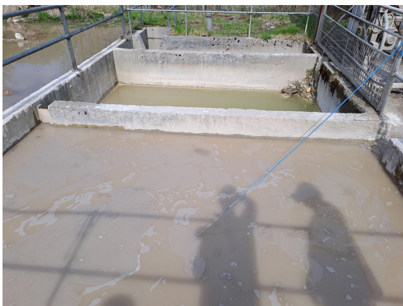
Figure 4 – The treatment pits at the time of the visit. No defects or issues observed.
