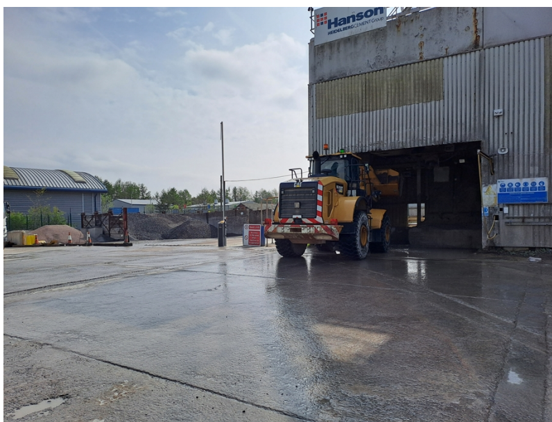
Figure 2 – General site conditions at the time of the visit.
