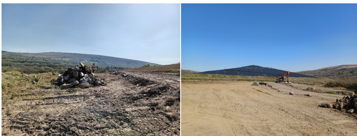
Image 4: Stockpiled restoration soils area - removed non-compliant material visible.
