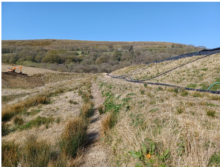
Image 1: Soil buttress - southern flank.
